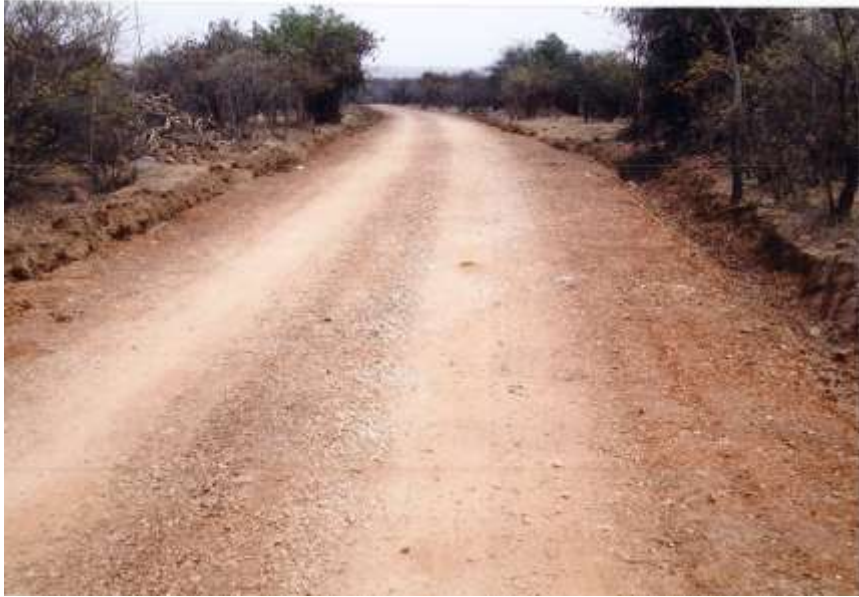
Maintenance of Road
