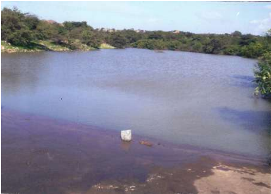
Check Dam at Kamalapura Block
